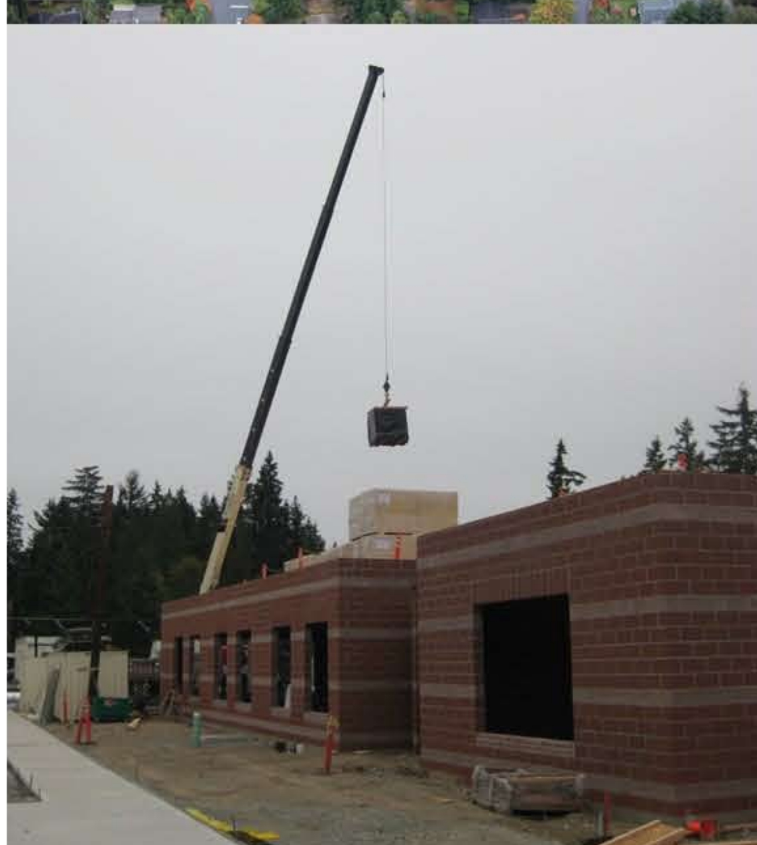
10/11/09 - Stockpiling the roofing material
