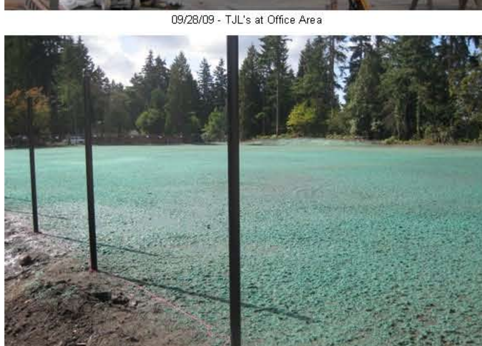
09/29/09 - Hydroseeding at Soccer Field
