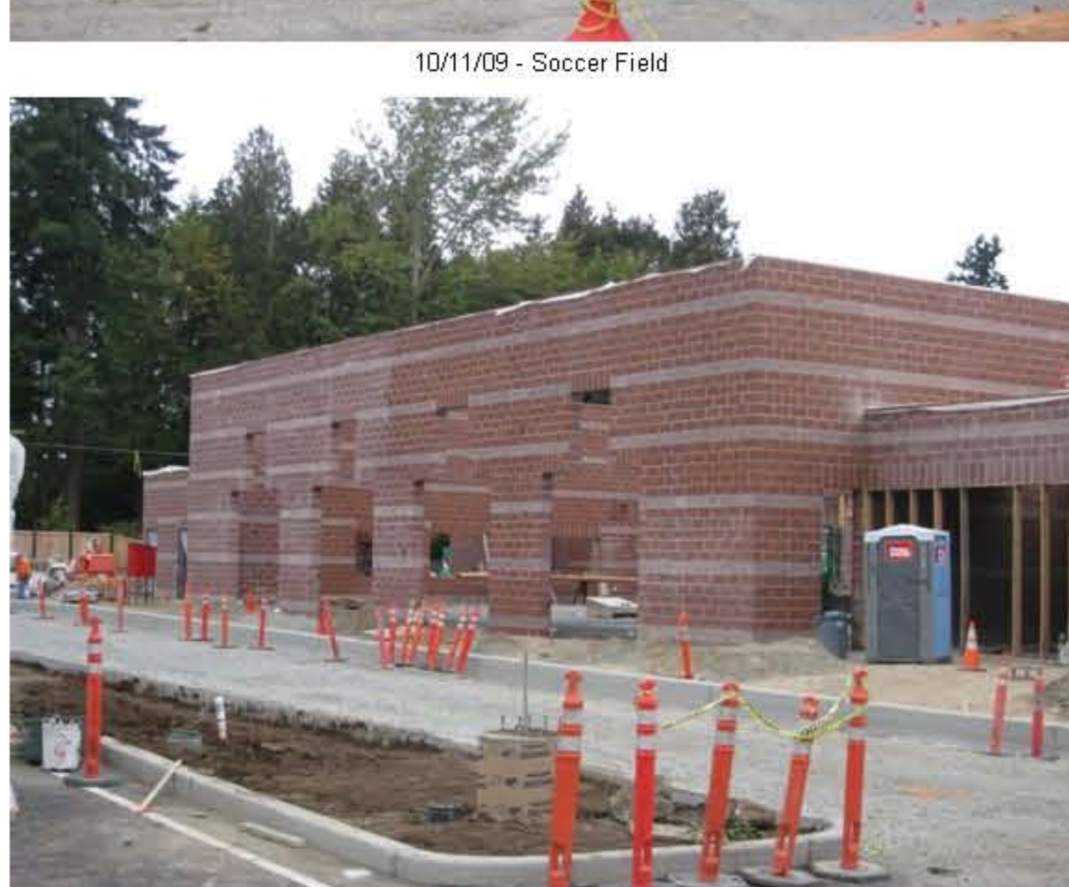
10/11/09 - South Elevation of Social Hall
