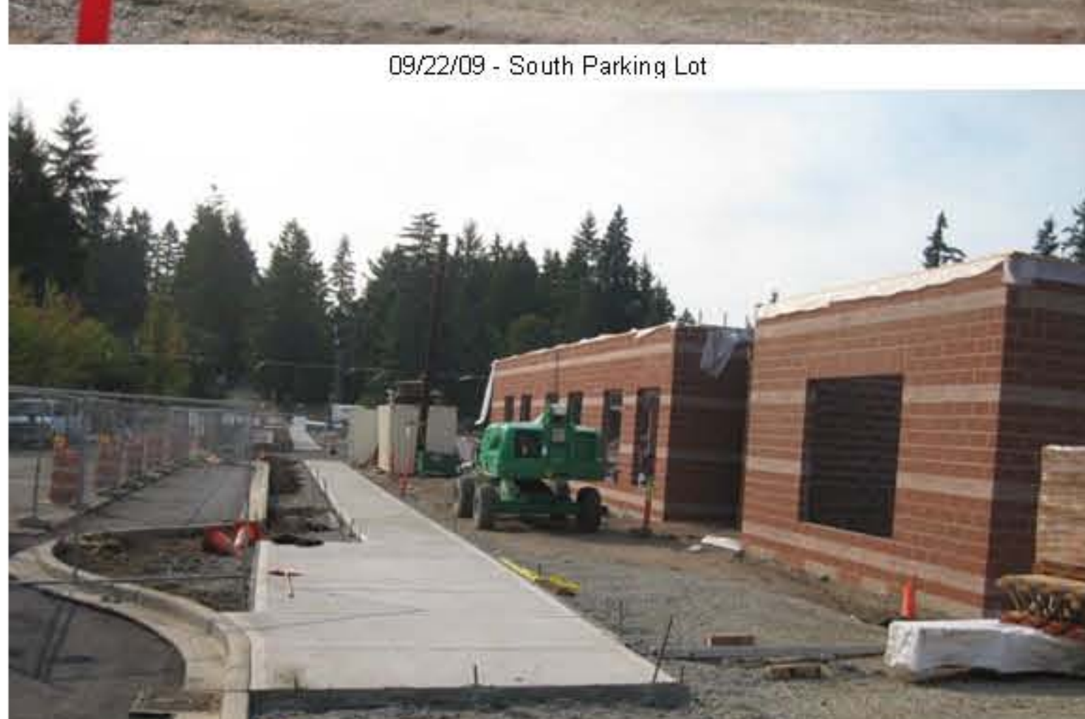
09/22/09 - Sidewalks and Curb/Gutter along 72nd Ave.
