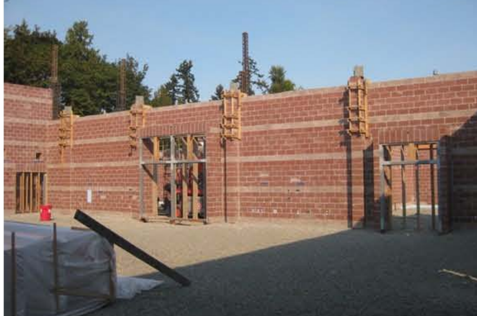
09/22/09 - North Elevation of Social Hall
