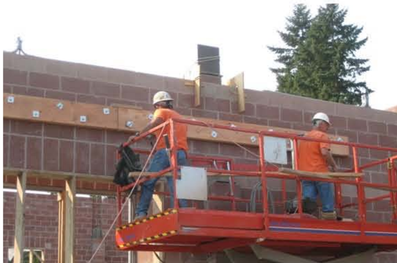
09/22/09 - Installing the ledger for the roof structure
