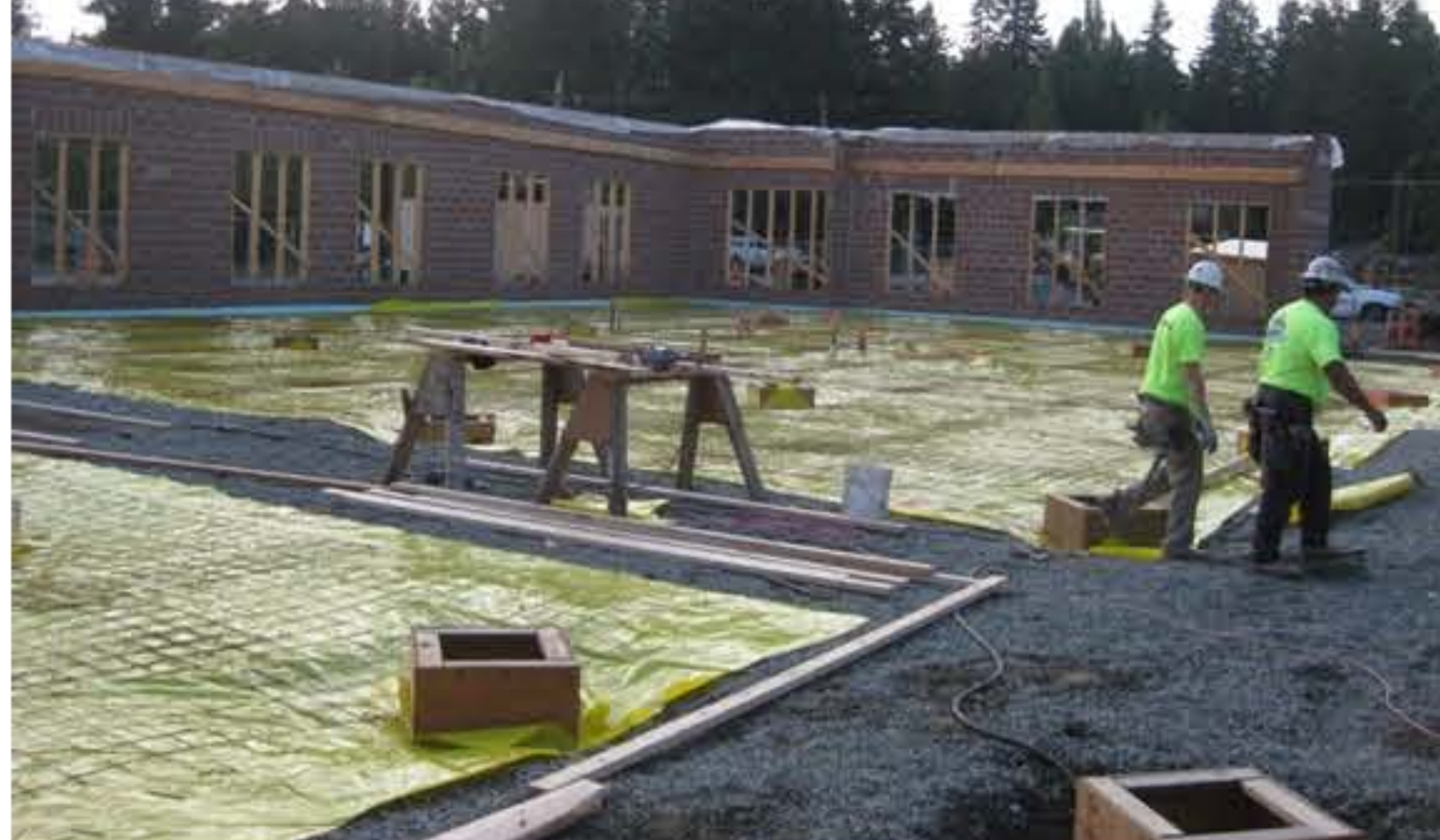
09/16/09 - Installing vapor barrier for our 1st slab pour
