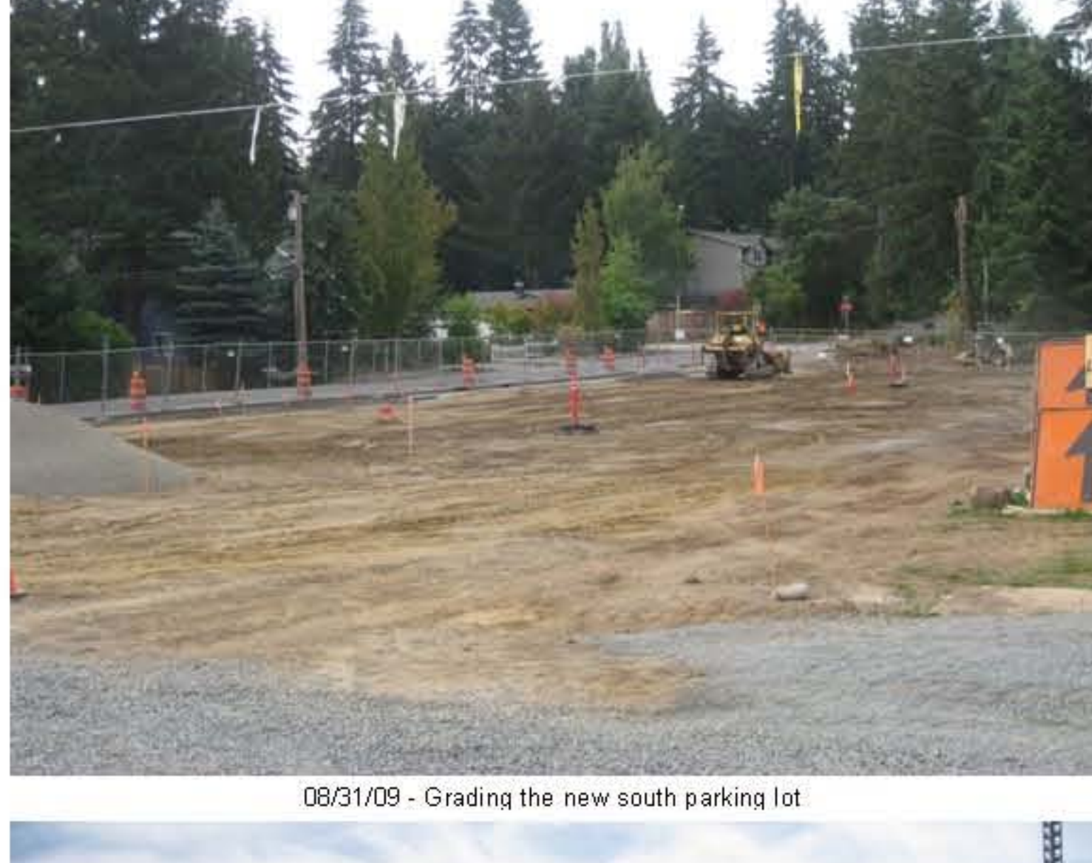
08/31/09 - Grading the new south parking lot
