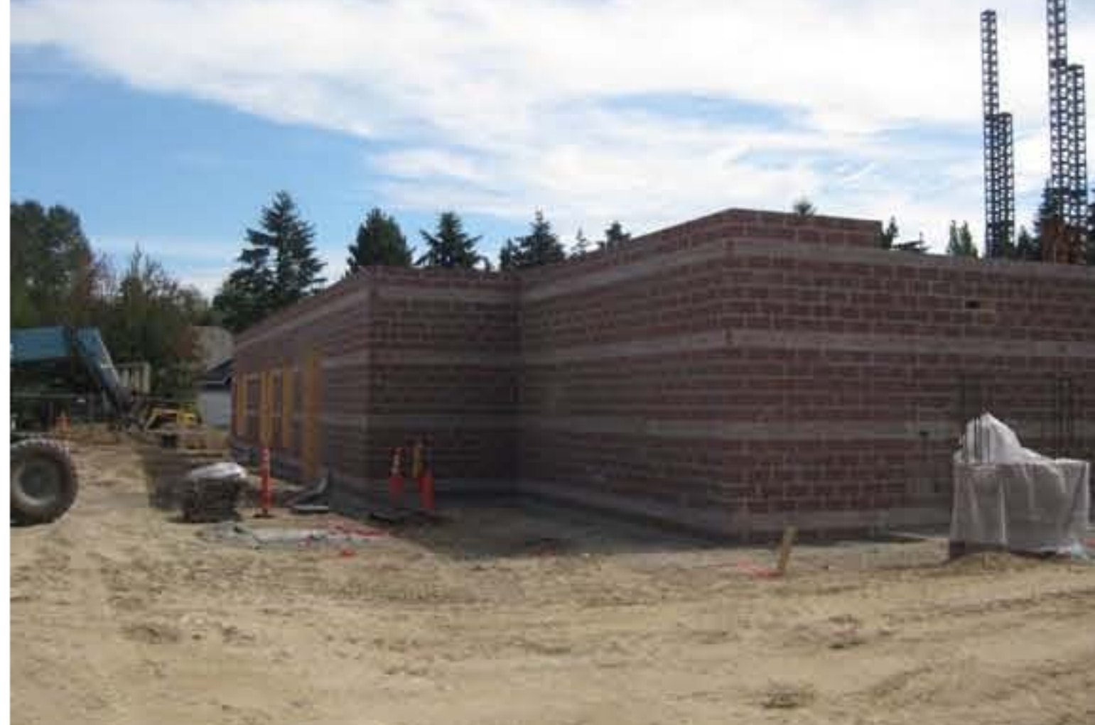
09/03/09 - CMU complete along the north side of the building
