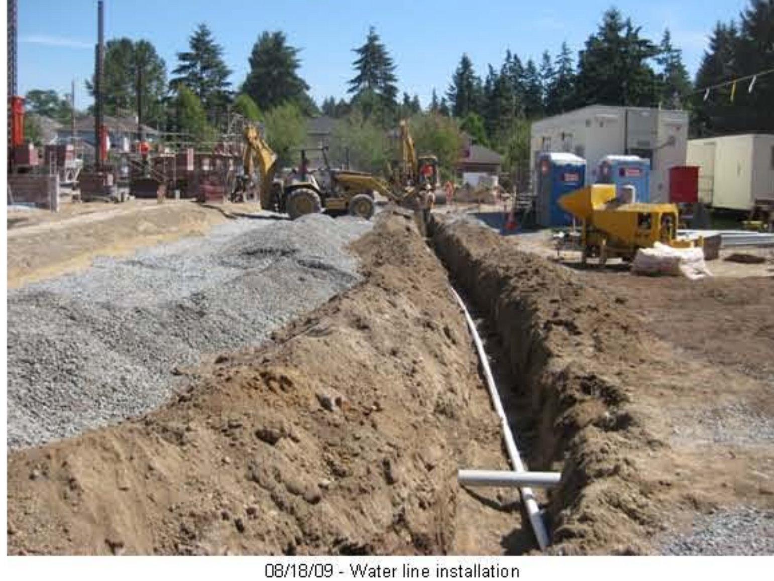
08/18/09 - Water line installation
