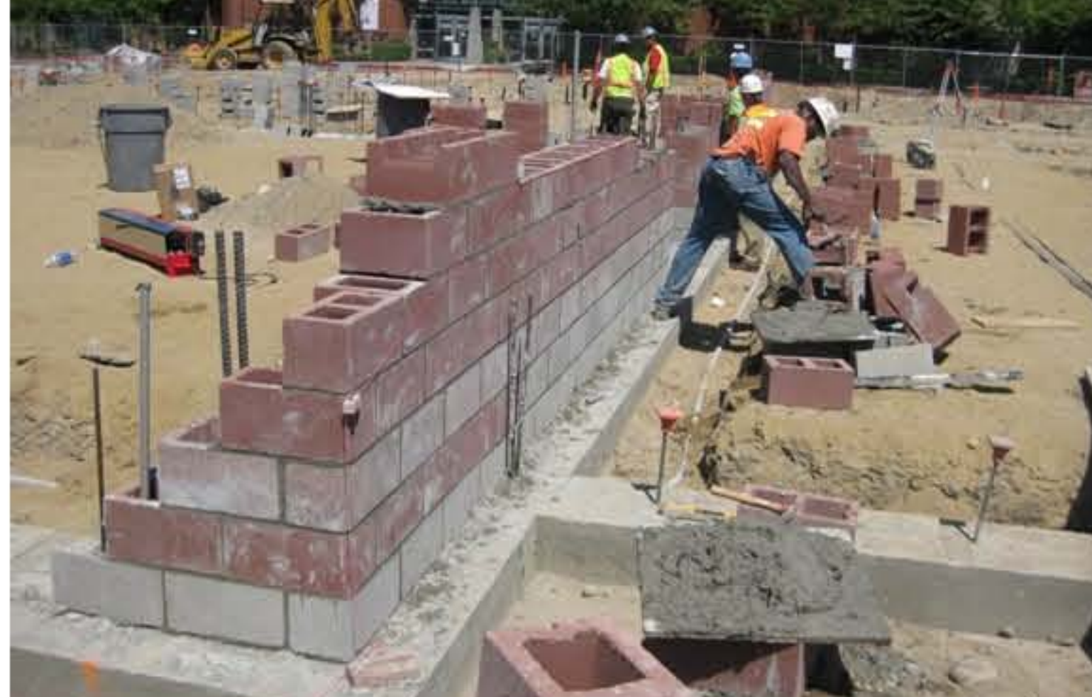
07/21/09 - First day of laying CMU block
