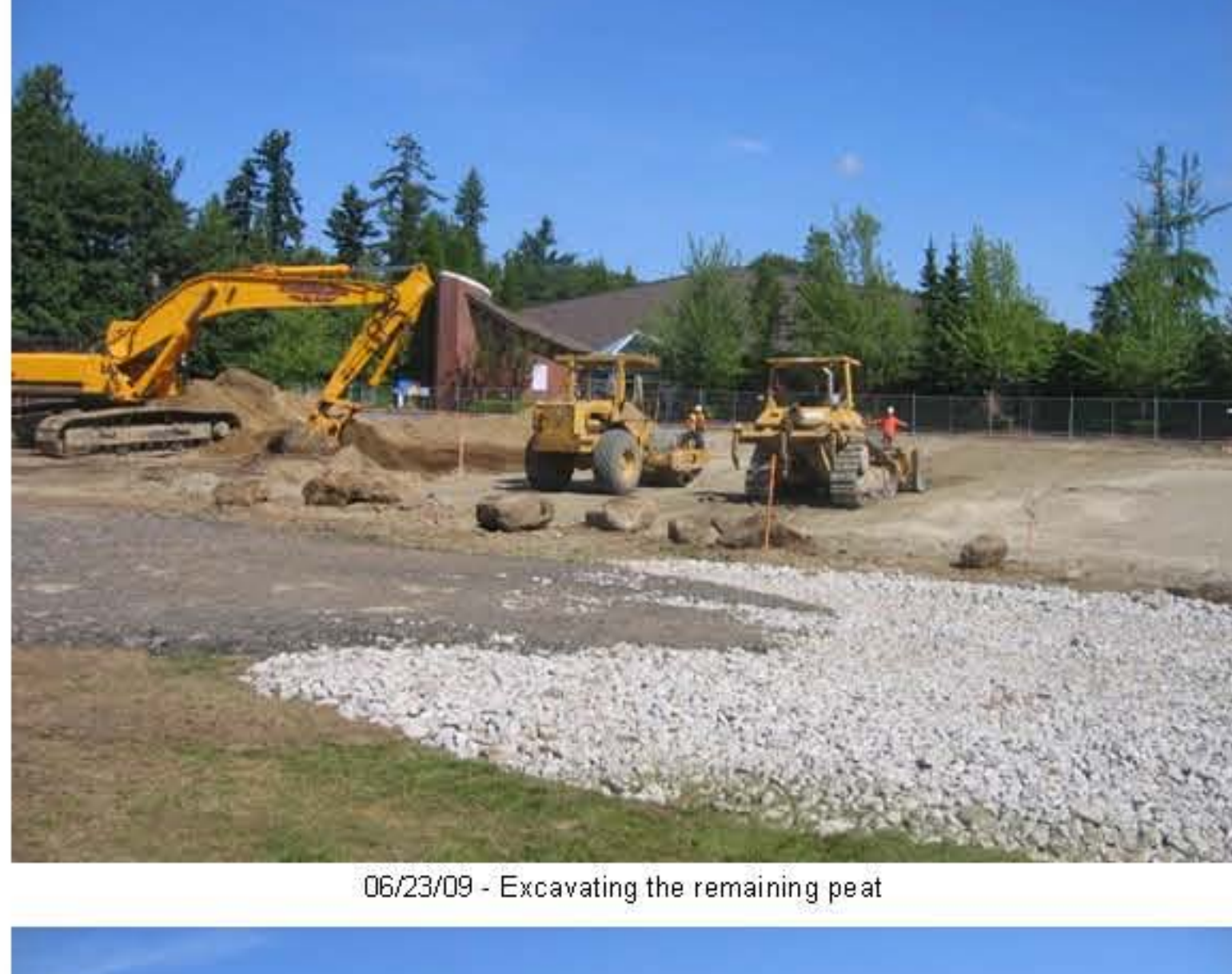
06/23/09 - Excavating the remaining peat
