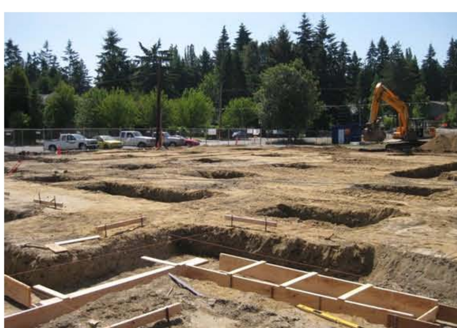
06/29/09 - Footing Formwork
