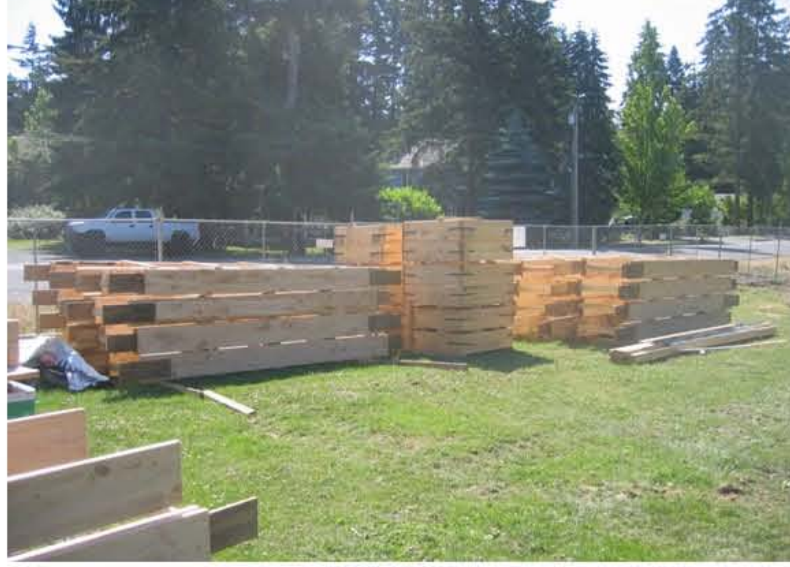
06/23/09 - Pre-built footing forms
