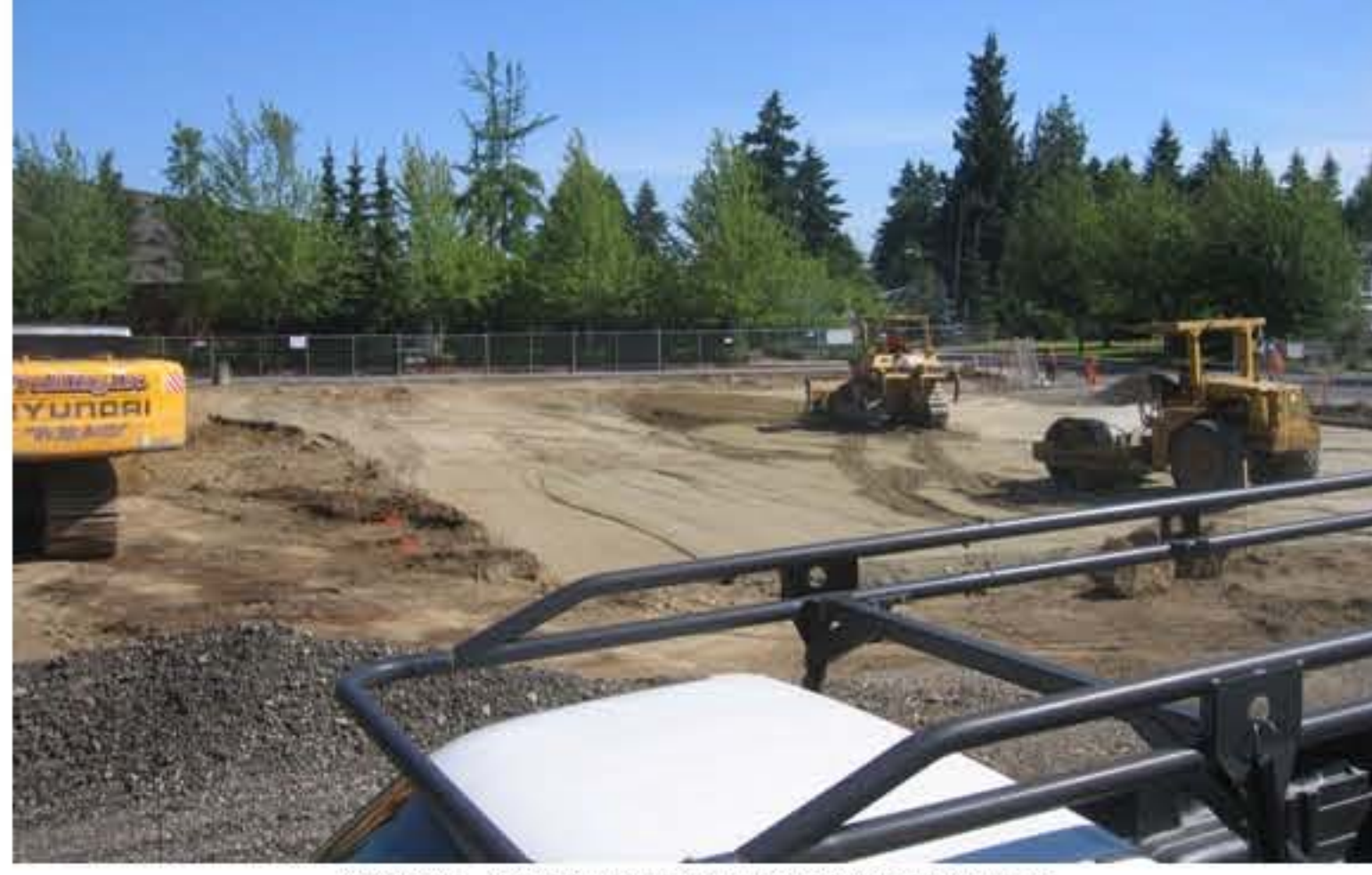
06/23/09 - Grading & compacting the building pad
