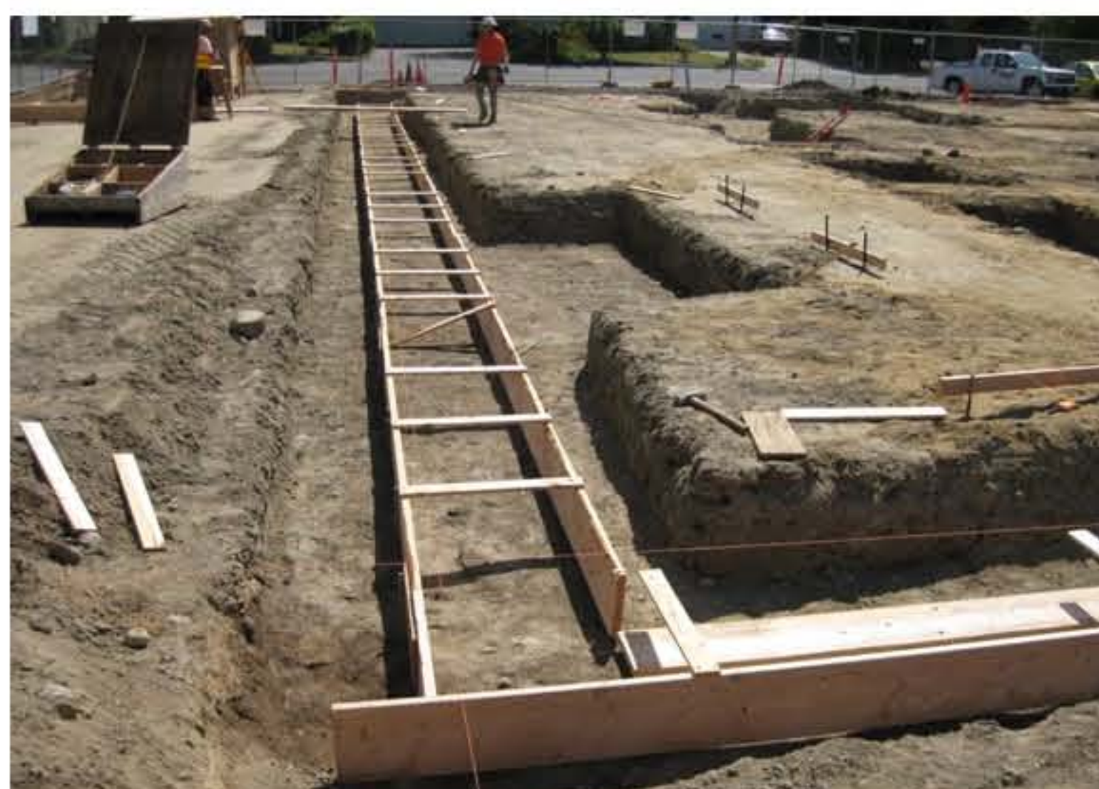
06/29/09 - Footing Formwork
