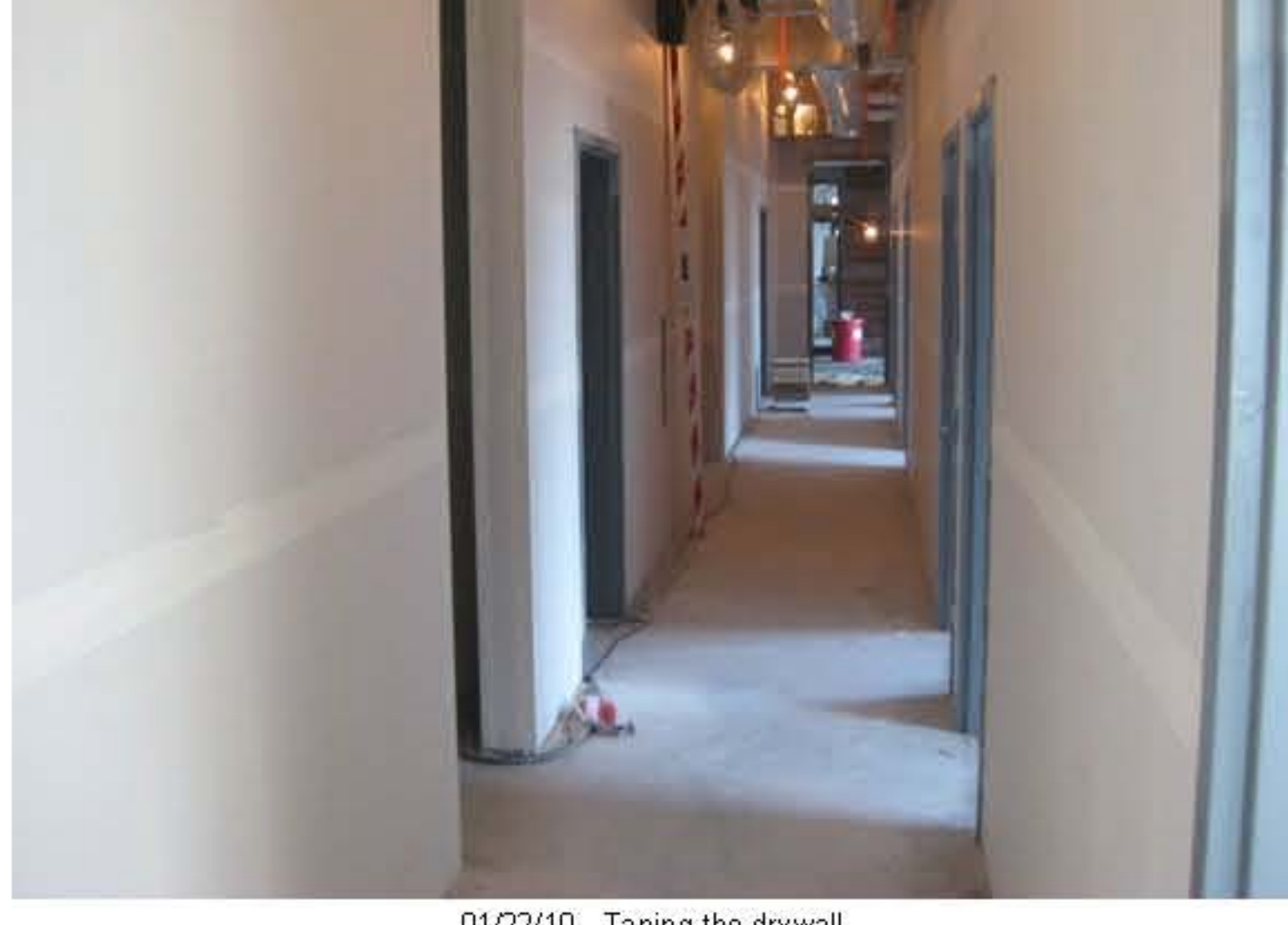
01/22/10 - Taping the drywall
