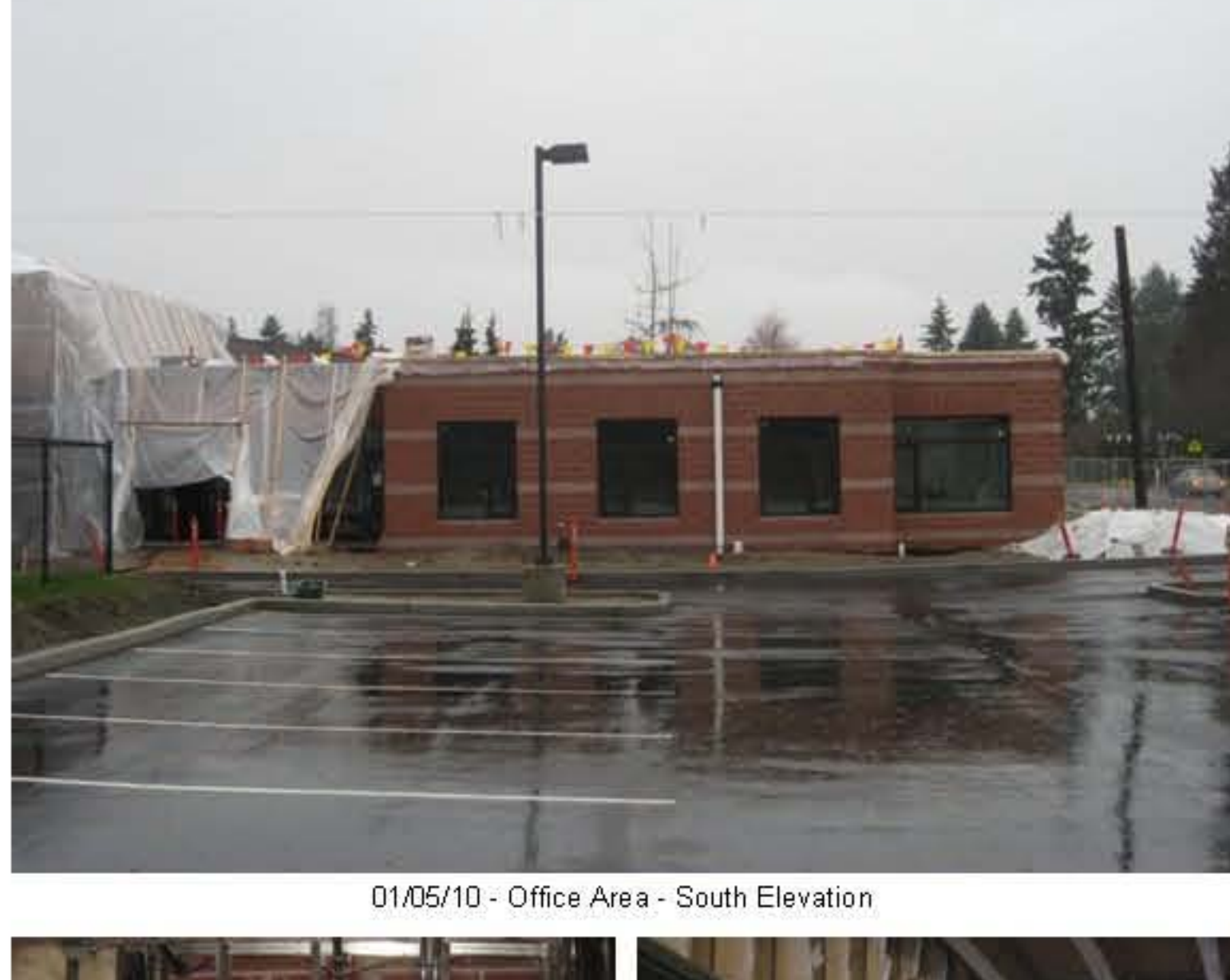
01/05/10 - Office Area - South Elevation
