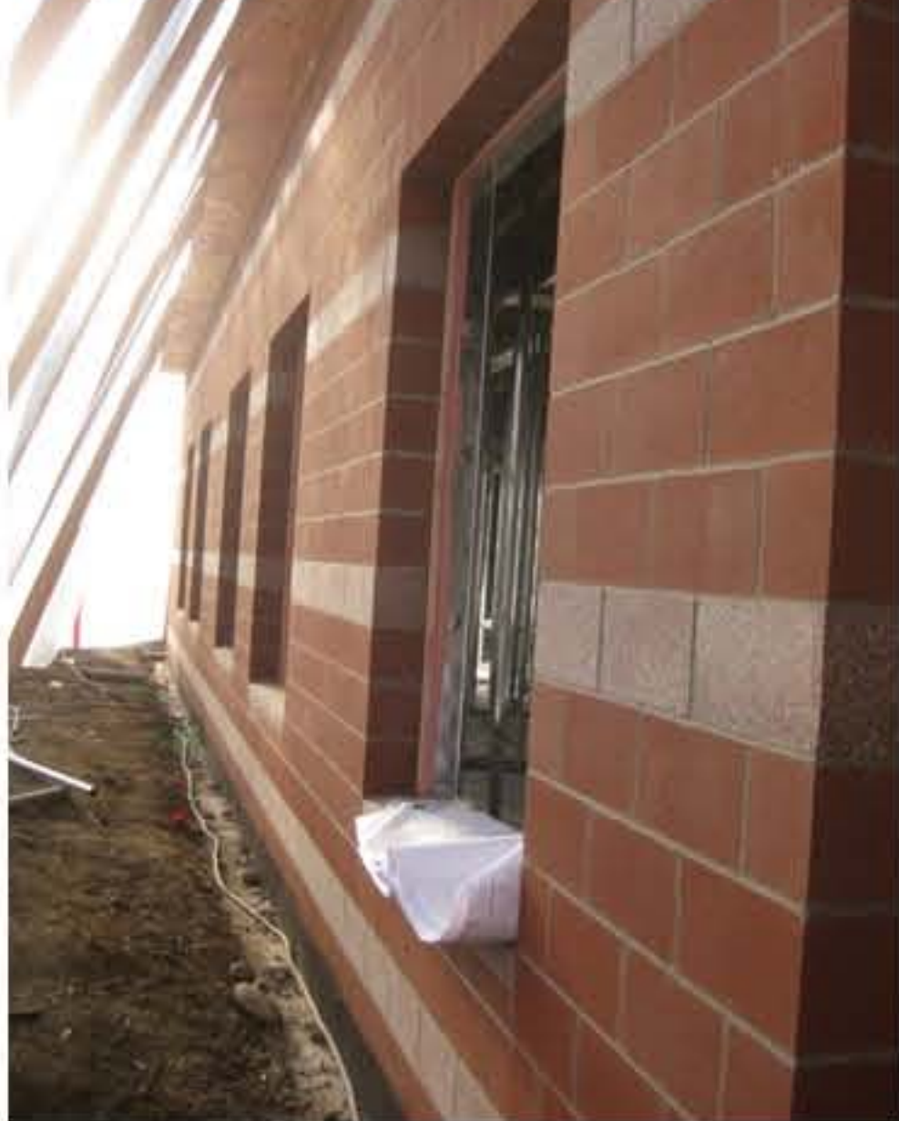
12/08/09 - Exterior East Elevation
