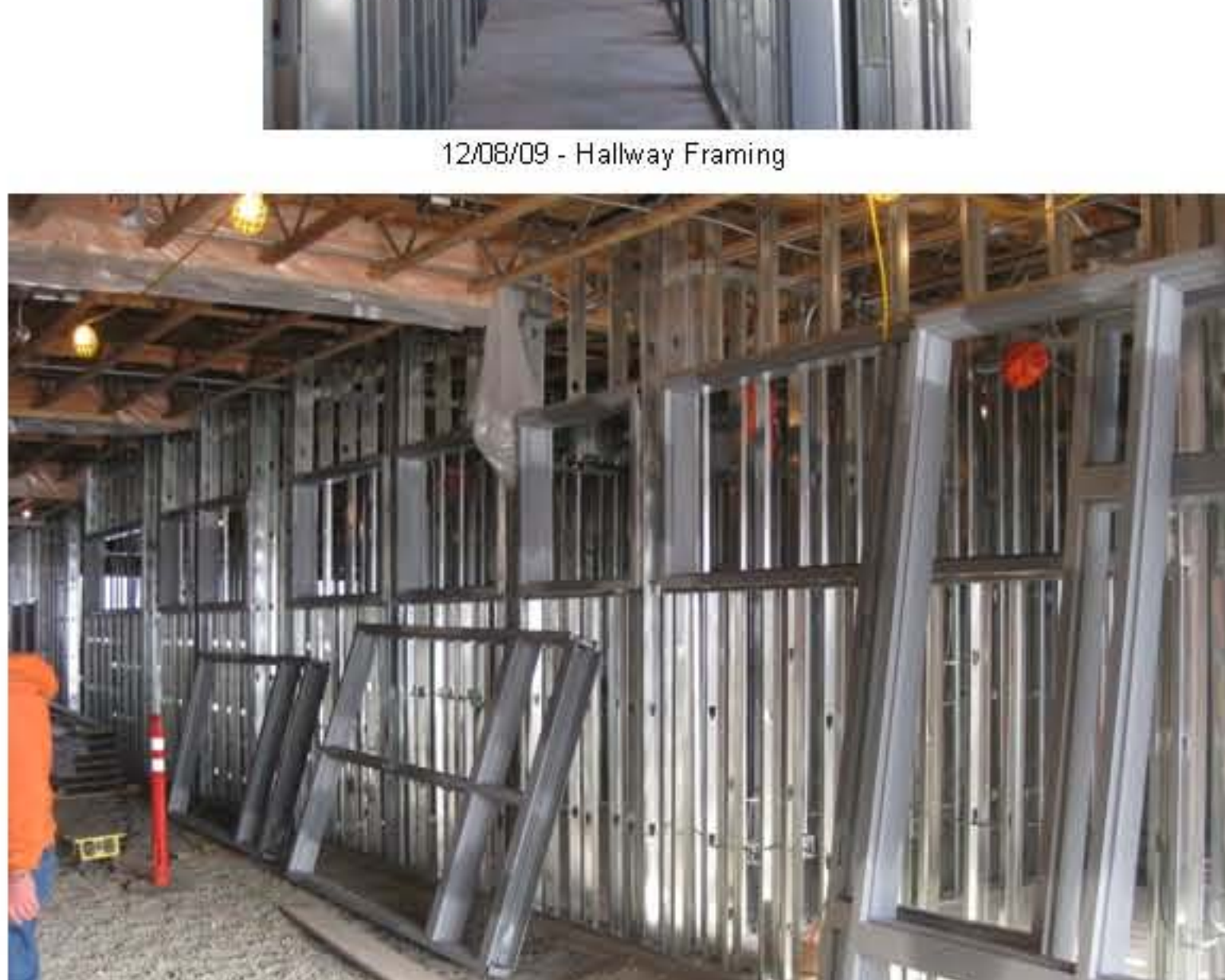
12/09/09 - Framing along South Entry hallway
