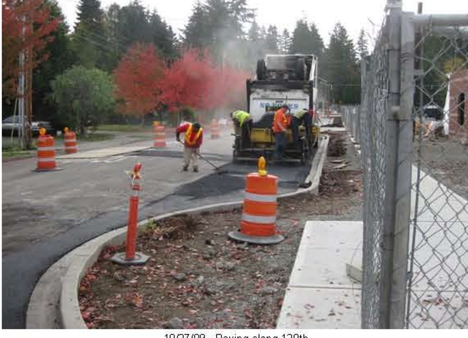
10/27/09 - Paving along 120th
