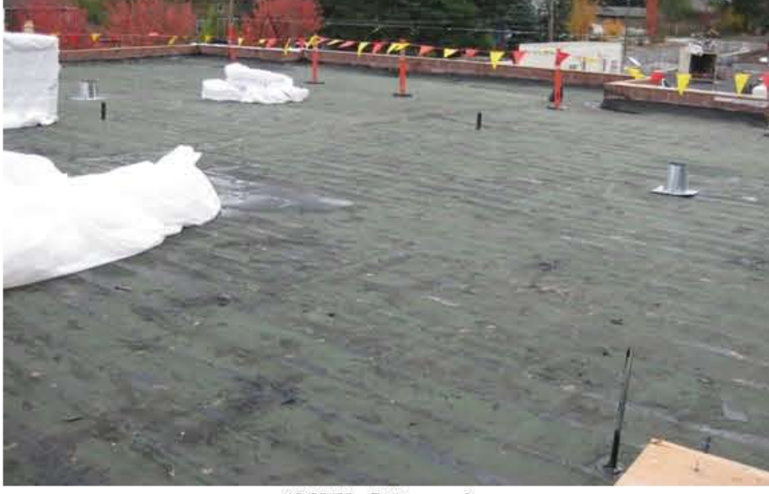
10/30/09 - Built-up roofing
