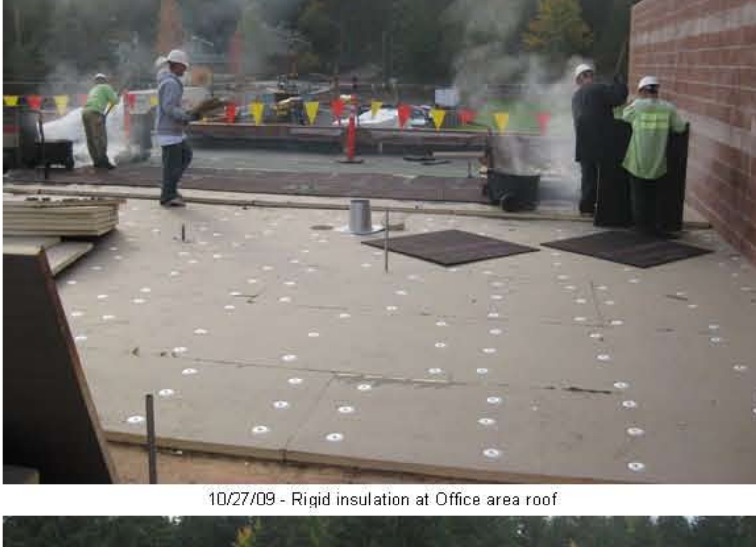
10/27/09 - Rigid insulation at Office area roof
