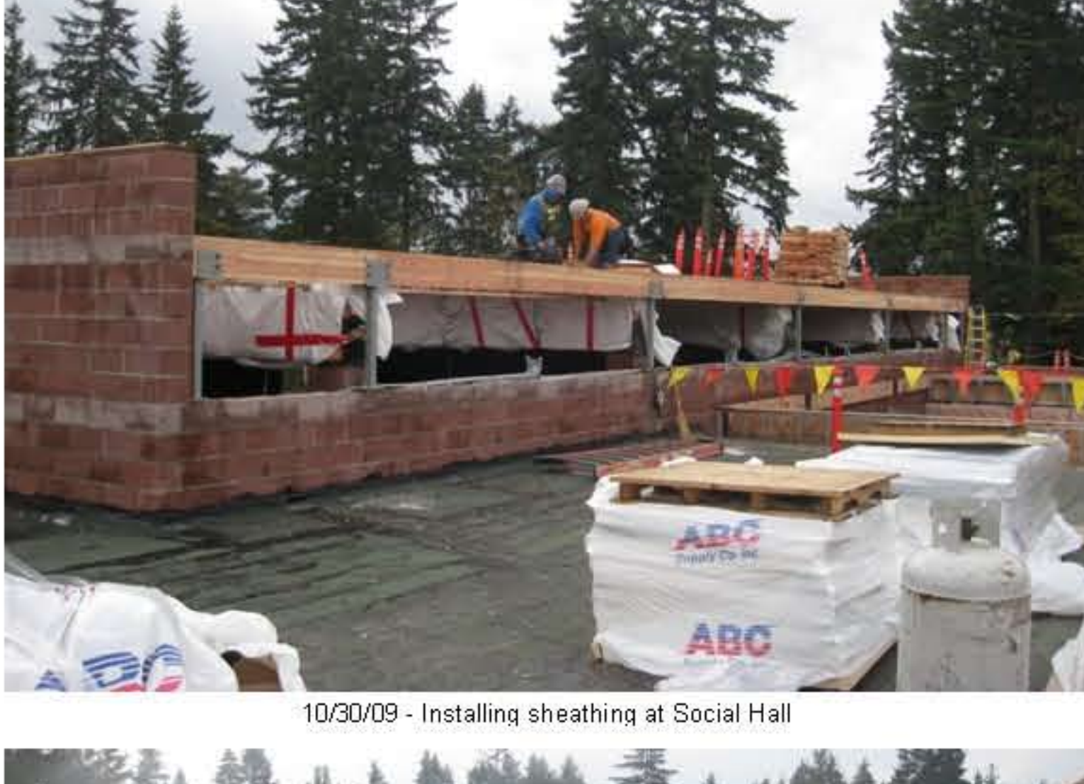
10/30/09 - Installing sheathing at Social Hall
