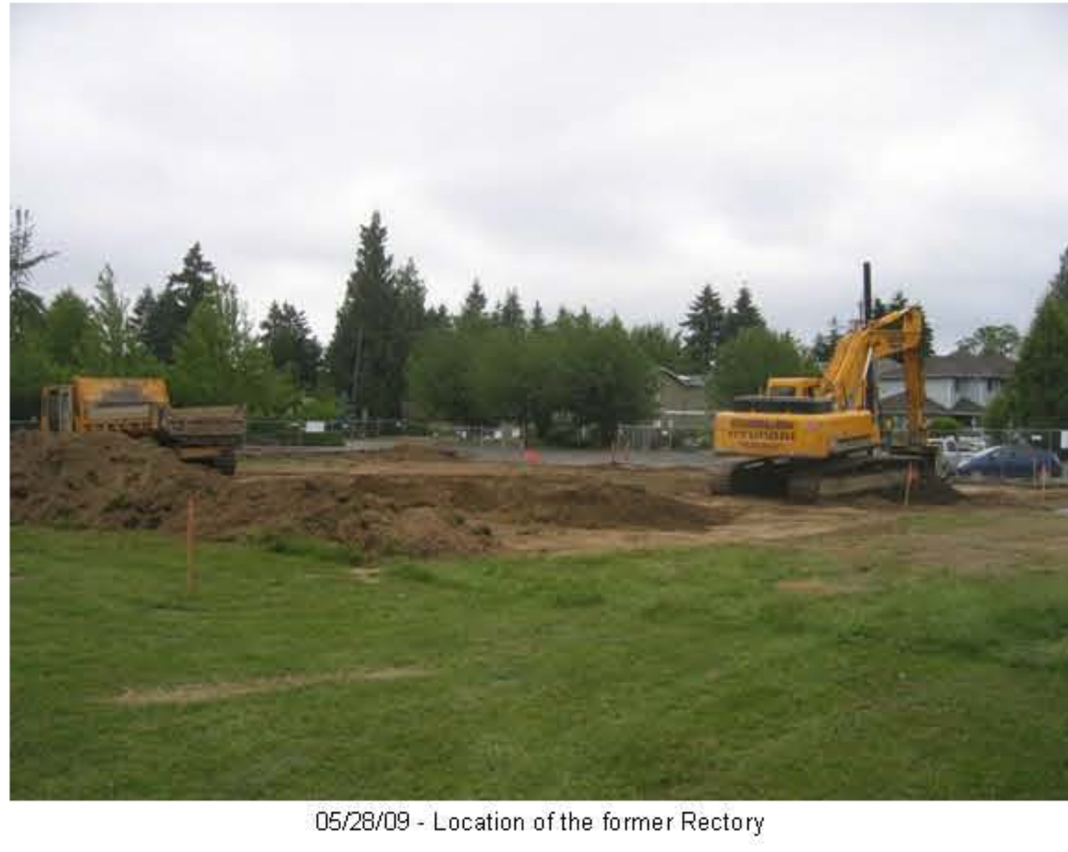
05/28/09 - Location of the former Rectory
